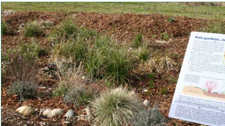
A rain garden, one of the effective components of LID (also illustrated at top of article).
